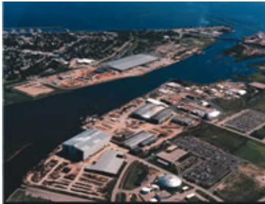
Marinette Marine Corporation’s ship construction facility in Marinette, WI.
