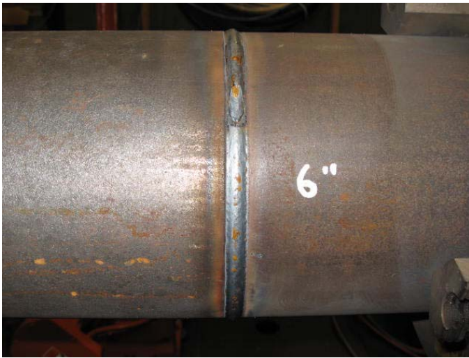
Figure 15. Photograph of the outside of a hybrid pipe weld produced at GD NASSCO, focused on the overlap region.
